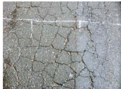
Photo 6. An example of several cracks on the surface
