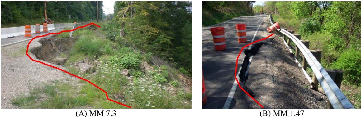
Figure 3. (A) Examples of rotational slides, affecting the embankment near SR-666 mile markers 7.3 (A) and 1.47 (B), respectively; extents outlined in red.
